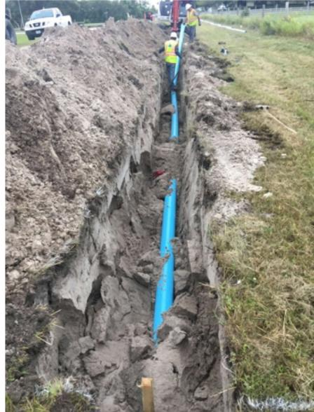
*R & A Road Boring LLC has begun the Water Line Improvements Project designed to loop water lines throughout the district. When complete, this project will eliminate numerous dead-ends in our water system.*
