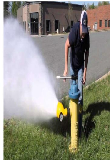
Flushing a fire hydrant also allows district workers to test its efficiency. Fire hydrants are, of course, used to fight fires, and the district needs to be sure that they will have enough water pressure and flow if the fire department were to need it.
