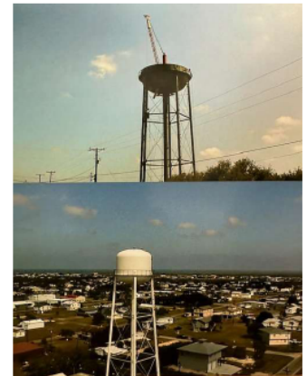
* Construction of Elevated Storage
